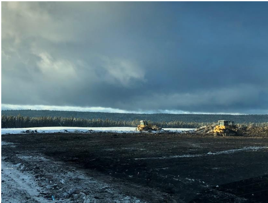
Figure 2 – Commencement of drilling site construction operations – December 4 2018
